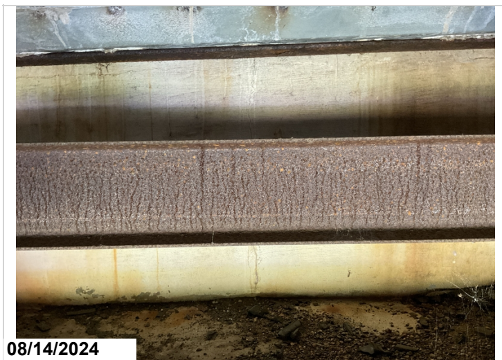
Bent 4 abutment, Cracking, CS2
