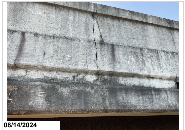
Concrete bridge railing, Both right and left sides, Cracking, CS2
