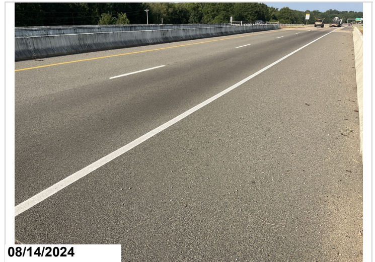
Polymer wearing surface photo
