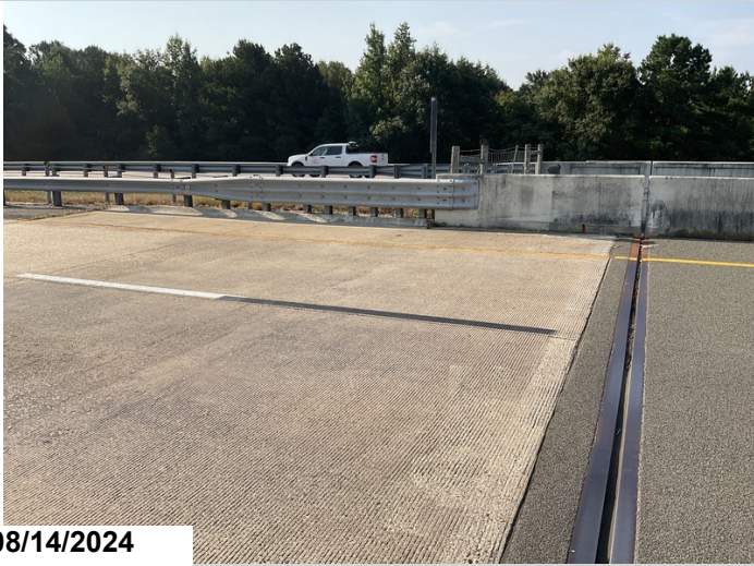
Bridge railing transition
