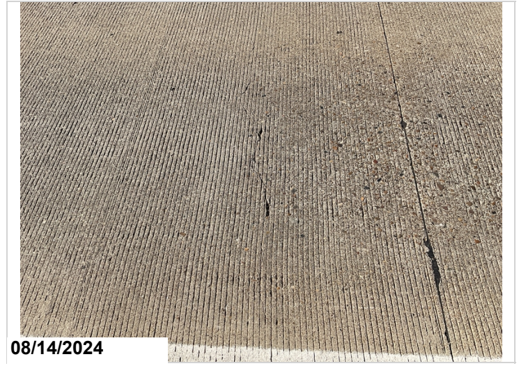
Beginning of bridge, Cracking in approach slab, CS2
