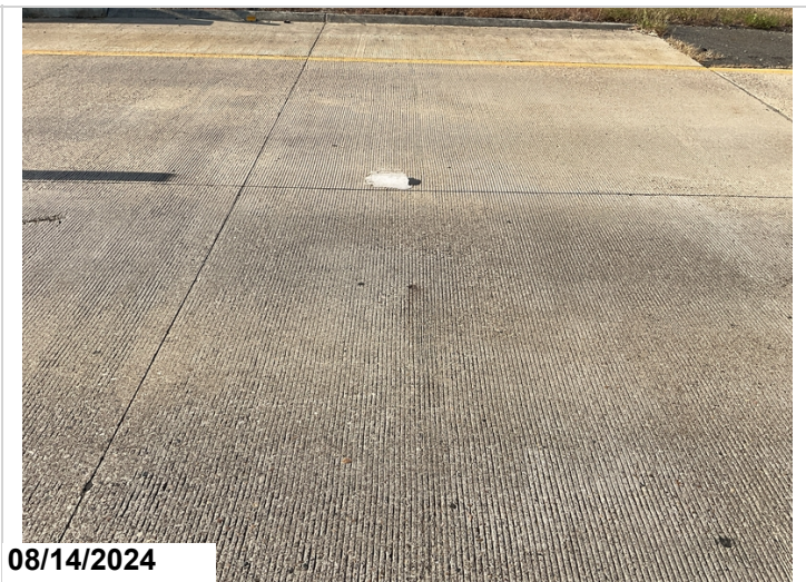
Beginning of bridge, Patched area, CS2
