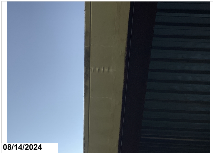
Deck, Undersurface, Efflorescence is found in various locations on both right and left overhangs, CS2
