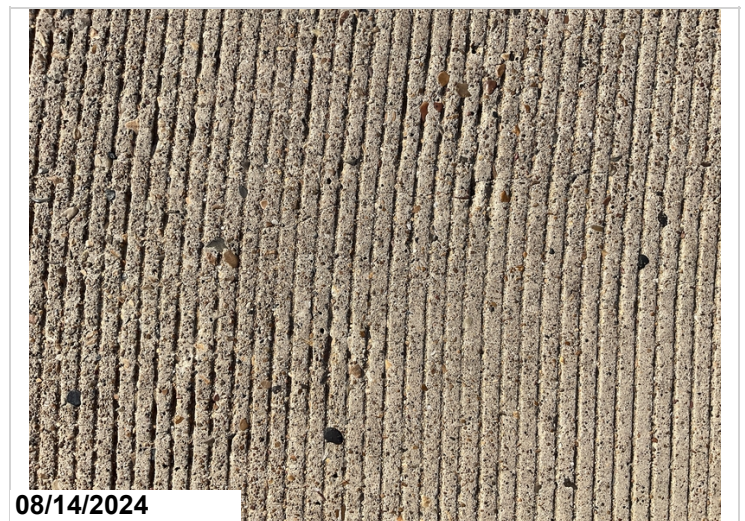
End of bridge, Cracking in approach slab, CS2
